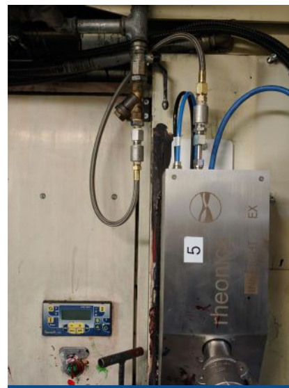
FIGURE 5. Adapter for in-line mounting of the sensor and including an auto wash system
